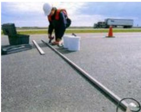
Figure 6: Piezoelectric sensor
