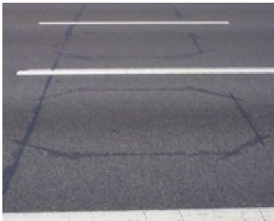
*Figure 1: inductive loop sensors*
