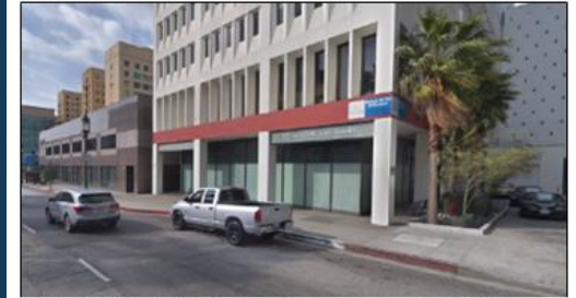
Recommendation 1A.1 Convert White Zone to Yellow Commercial Loading Zone (F) Source: Google Streetview
