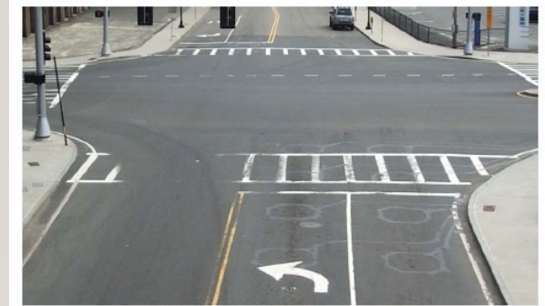
(b) Physical representation of loop detectors
