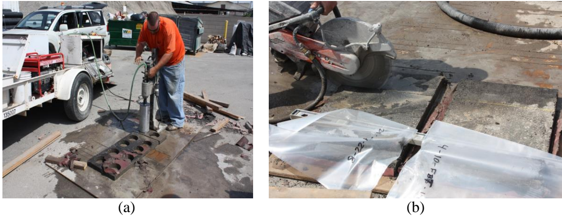
Figure 2. a) Coring SCB specimens and b) Sawing FBT specimens.
