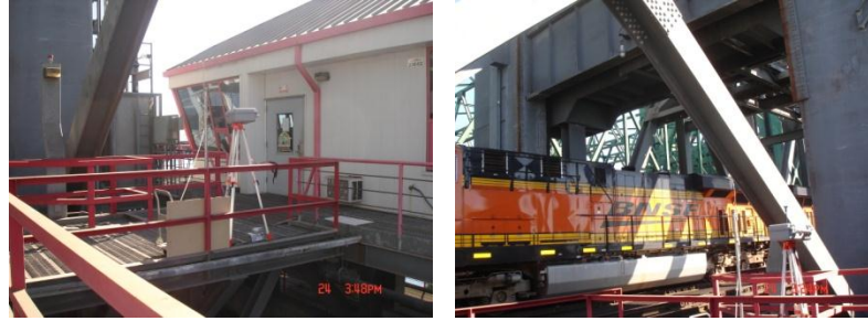
Figure 5. Field test measurements.
